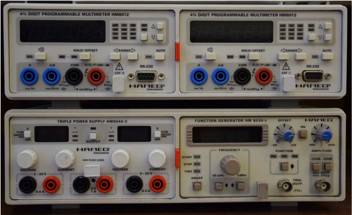
Figure 4. : The electrical instruments at the lab, without the oscilloscope
