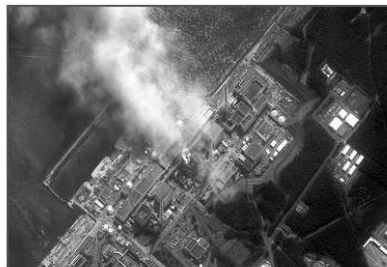
Fire at Fukushima Daiichi following earthquake and tsunami
